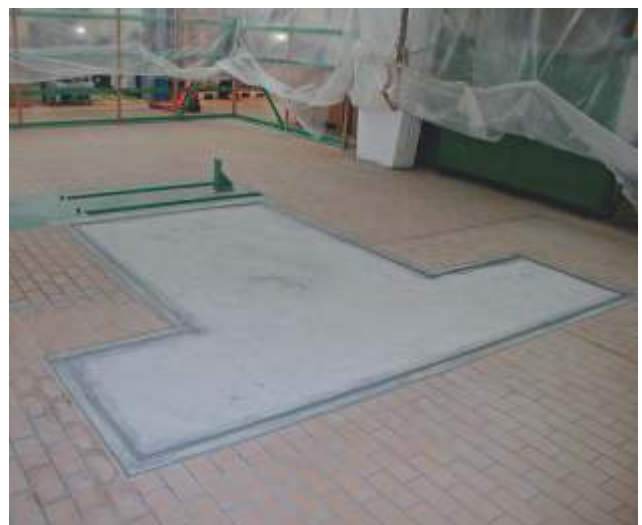
Cast foundation block
